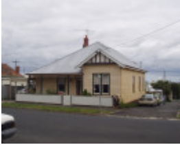
122 Maud Street, Geelong
