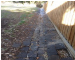
Bluestone drain Brisbane St and Ormond Rd
