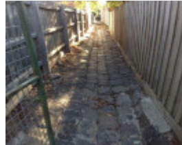
Bluestone drain Brisbane St and Ormond Rd
