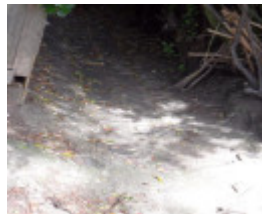
Brisbane St drain b
