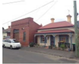
Ascot Vale Fire Station and residence (former)
