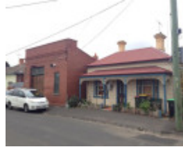
Ascot Vale Fire Station and residence (former)
