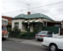
Crown St 17 house
