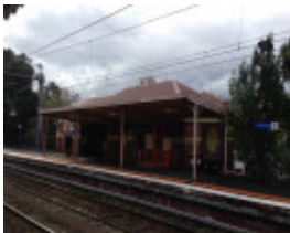
Newmarket Railway Station Up side building
