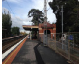
Newmarket Railway Station Down side building
