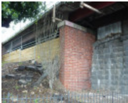
Racecourse Road Bluestone bridge abutment west side
