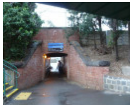
Newmarket Railway Station Pedestrian Subway east side
