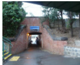
Newmarket Railway Station Pedestrian Subway east side
