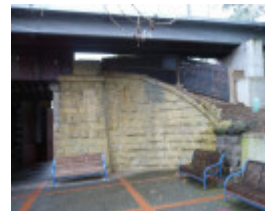
Racecourse Road Railway Bridge abutment east side
