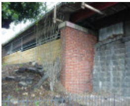
Racecourse Road Bluestone bridge abutment west side
