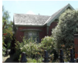
The Crescent 59 a
