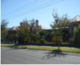
Ardmillan Road Precinct north side nos. 28 to 30
