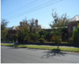
Ardmillan Road Precinct north side nos. 28 to 30
