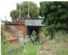
Grice Cr railway bridge.JPG
