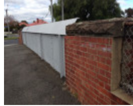
Road over rail bridge between Grice Cres and Napier St
