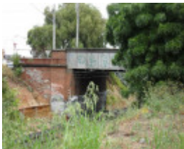
Grice Cr railway bridge.JPG
