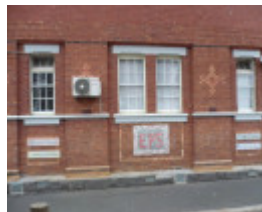
Essendon Primary School No.483 1922 block showing earlier nineteenth century windows
