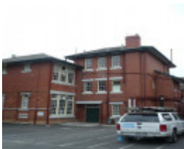
Essendon Primary School No.483 1922 block
