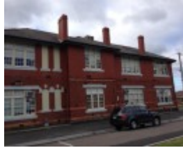
Essendon Primary School No.483 1922 school
