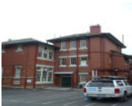
Essendon Primary School No.483 1922 block
