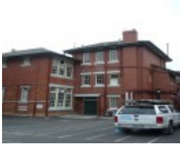
Essendon Primary School No.483 1922 block
