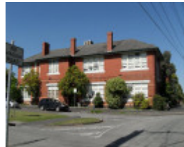
Essendon Primary School No.483 1922 school west elevation
