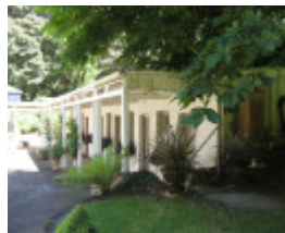
PROV H2204_Duneira_service block_19 Jan 09 96
