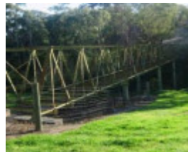
2011, Plenty River pipe bridge.gif
