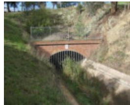
2011, brickwork to tunnel 4.gif
