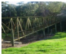
2011, Plenty River pipe bridge.gif
