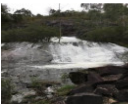
2017, base of spillway.jpg
