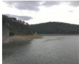
2017 looking north to outlet tower.jpg
