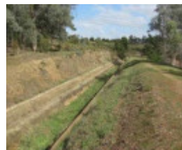
2011, decommissioned aqueduct, central section.gif
