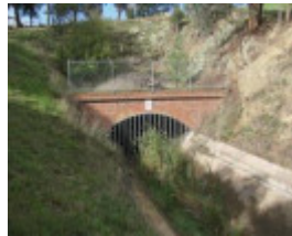
2011, brickwork to tunnel 4.gif
