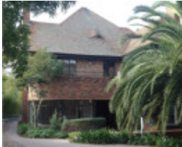
420-424 Punt Road, South Yarra
