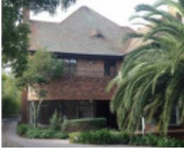
420-424 Punt Road, South Yarra
