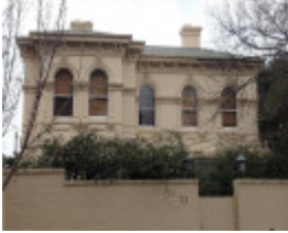
21 William Street, South Yarra (prior to removal of verandah)
