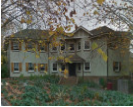
9 Linlithgow Road, Toorak
