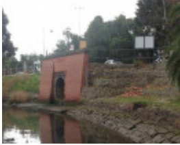
Holmes Road drain outlet
