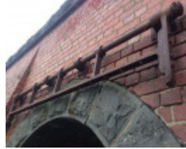
Holmes Road drain outlet
