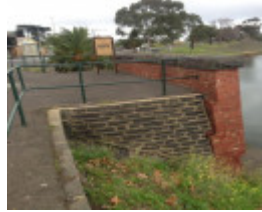
Holmes Road drain outlet
