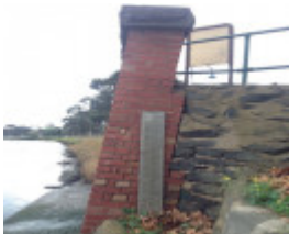
Holmes Road drain outlet
