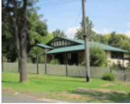
Subject property as seen from Harker Street
