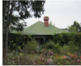
View of the north elevation and return verandah
