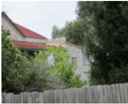
North elevation and verandah enclosure to the rear
