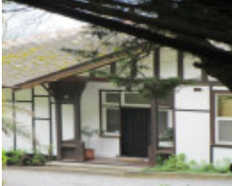
Detail of entrance to property
