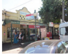
Another view of the subject property, in the commercial streetscape context.
