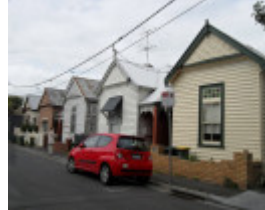
Timber cottages, south side of Bliss Street
