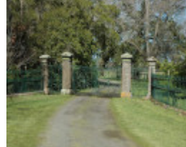
Illustration 3 Gates at Killarney, Dunnstown, 1901 have a similar scale and layout but differ in detail and cast iron pattern. They were designed by George Clegg, architect of Ballarat, who had also designed James Coghlan's home in Ballarat in 1888 and if
