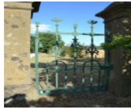
Photo 2 Detail of Pedestrian Gate.jpg
