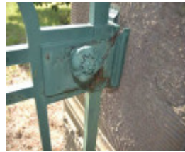
Photo 3 Detail of lock and cast iron handle.jpg
