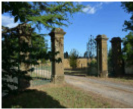
Photo 1 Gate Posts and Cast Iron Gates.jpg
