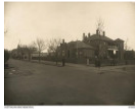
Former Red Cross Rest House
