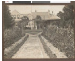
Former Red Cross Rest House
