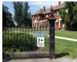
Former Red Cross Rest House
