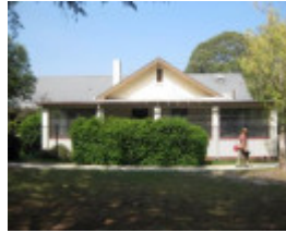
Former Red Cross Rest House
