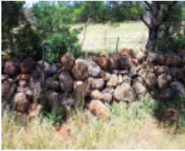
Dry Stone Wall C49
