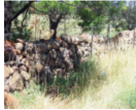
Dry Stone Wall C49
