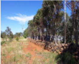
Dry Stone Wall C50
