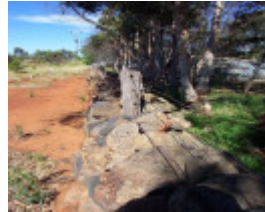
Dry Stone Wall C50
