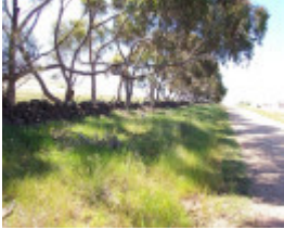
Dry Stone Wall C52
