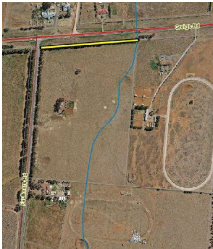
Dry Stone Wall C61
