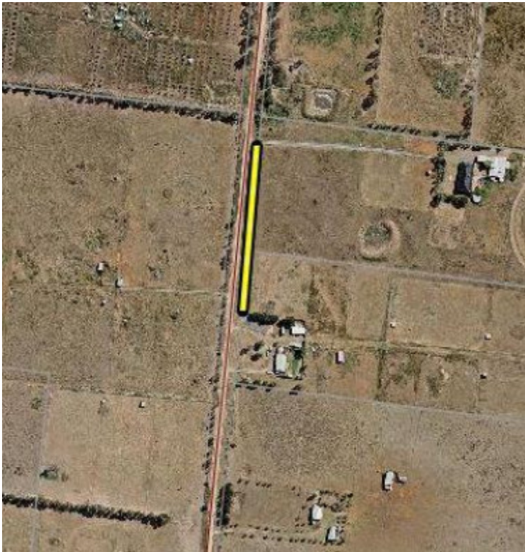
Dry Stone Wall G91
