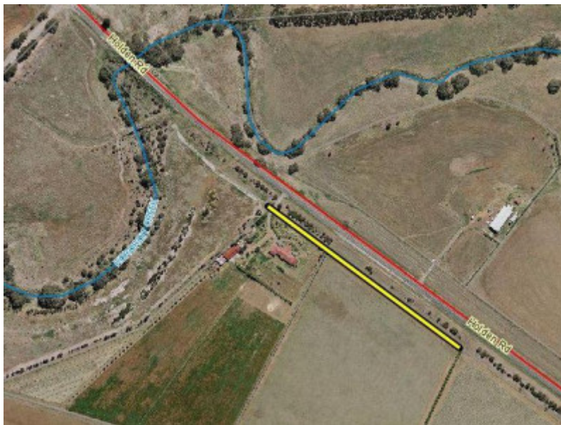
Dry Stone Wall R242
