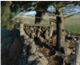
Dry Stone Wall R194
