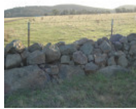
Dry Stone Wall R194
