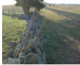
Dry Stone Wall R194
