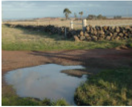
Dry Stone Wall R194
