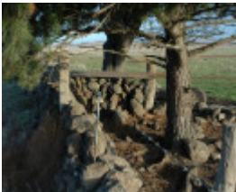
Dry Stone Wall R194
