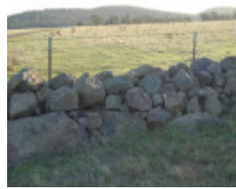
Dry Stone Wall R194
