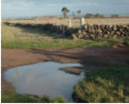
Dry Stone Wall R194
