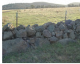
Dry Stone Wall R194
