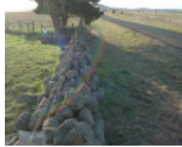
Dry Stone Wall R194
