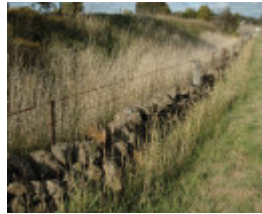
Dry Stone Wall R245
