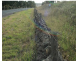
Dry Stone Wall R245
