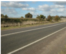
Dry Stone Wall R245
