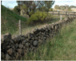
Dry Stone Wall R245
