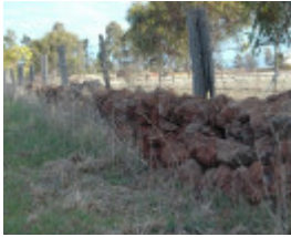
Dry Stone Wall R247
