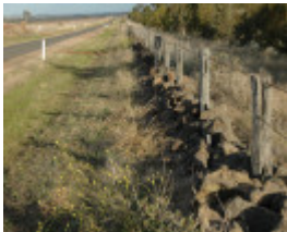
Dry Stone Wall R247
