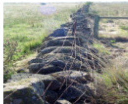
Dry Stone Wall B115
