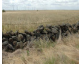
Dry Stone Wall B115
