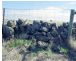
Dry Stone Wall B115
