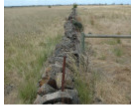
Dry Stone Wall B115
