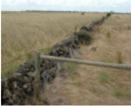
Dry Stone Wall B115
