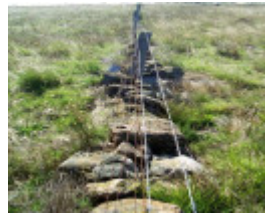
Dry Stone Wall B116
