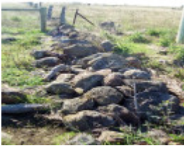
Dry Stone Wall B116
