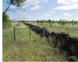
Dry Stone Wall B121
