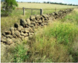
Dry Stone Wall B121
