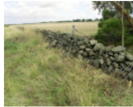
Dry Stone Wall B123
