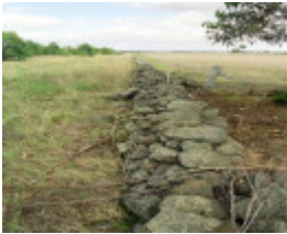
Dry Stone Wall B123
