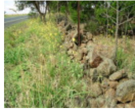
Dry Stone Wall B124
