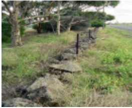
Dry Stone Wall B124
