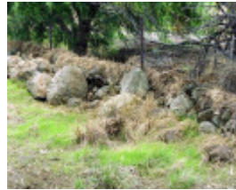
Dry Stone Wall B125
