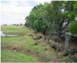
Dry Stone Wall B125
