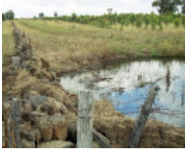
Dry Stone Wall B126
