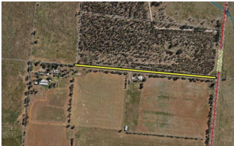
Dry Stone Wall B126
