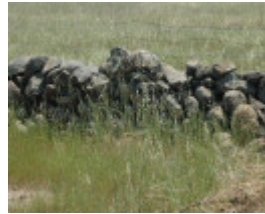
Dry Stone Wall B169
