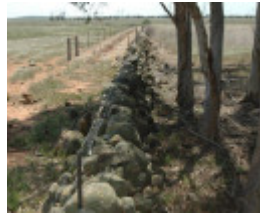
Dry Stone Wall B170
