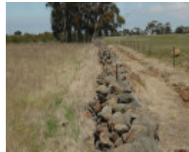
Dry Stone Wall B170
