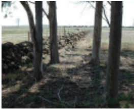
Dry Stone Wall B170
