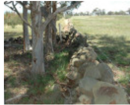
Dry Stone Wall B170
