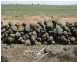
Dry Stone Wall B170
