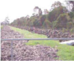
Dry Stone Wall B45
