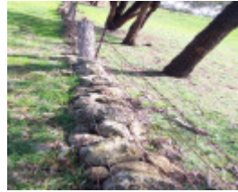
Dry Stone Wall B46
