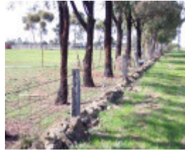
Dry Stone Wall B46
