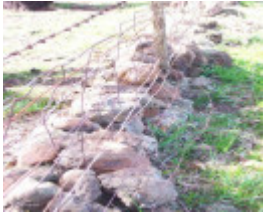
Dry Stone Wall B46
