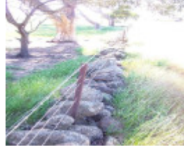
Dry Stone Wall G85
