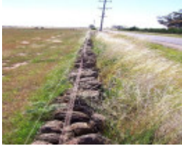
Dry Stone Wall G85
