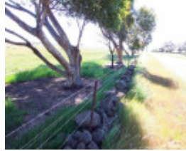
Dry Stone Wall G85
