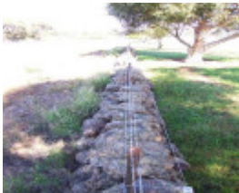
Dry Stone Wall G85
