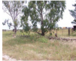
Dry Stone Wall C71
