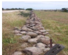
Dry Stone Wall C71
