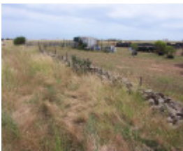
Dry Stone Wall C71
