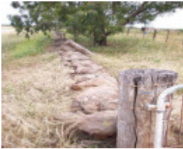
Dry Stone Wall C71
