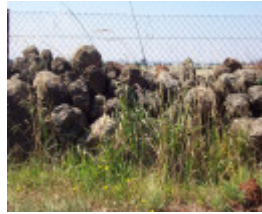
Dry Stone Wall D81
