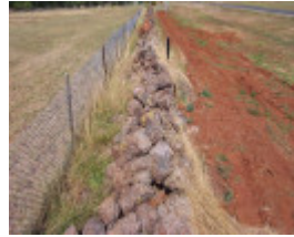
Dry Stone Wall D81
