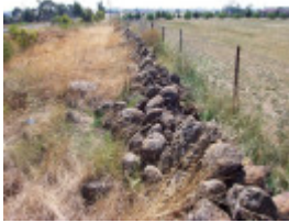
Dry Stone Wall D81
