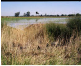
Dry Stone Wall J132
