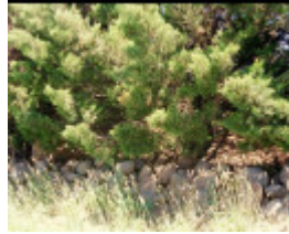
Dry Stone Wall J132
