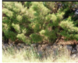
Dry Stone Wall J132
