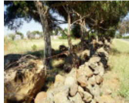
Dry Stone Wall J133
