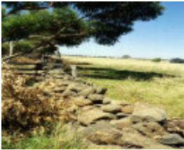
Dry Stone Wall J134
