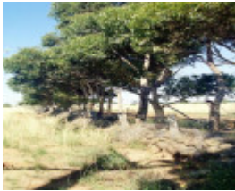
Dry Stone Wall J143
