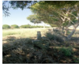
Dry Stone Wall J143
